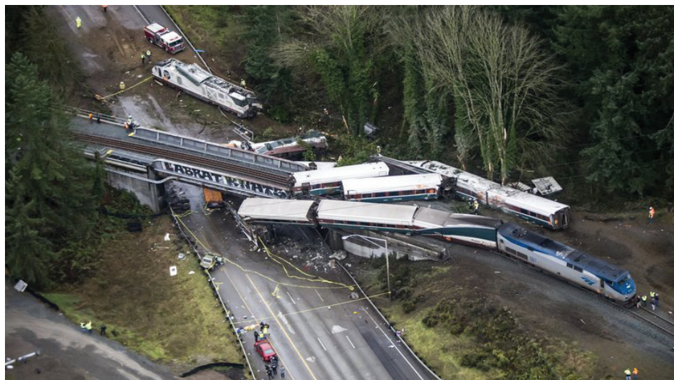
Amtrak Cascades Train 501 derailed on December 18, 2017.
