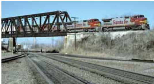
A flyover near Kansas City, akin to those to be built around Chicago as part of CREATE (Courtesy The Viewliner Limited blog)
